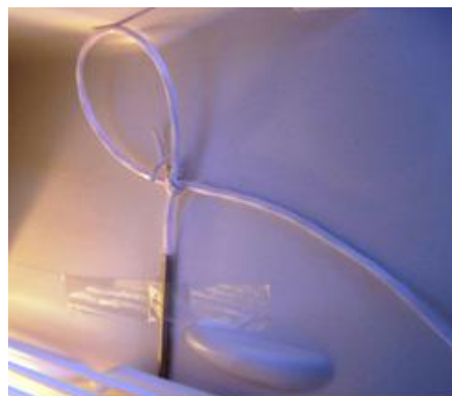
Figure 3: Best practise – The sensor cable is not bend behind the Teflon seal and the loop acts as a strain relief for the cable.
