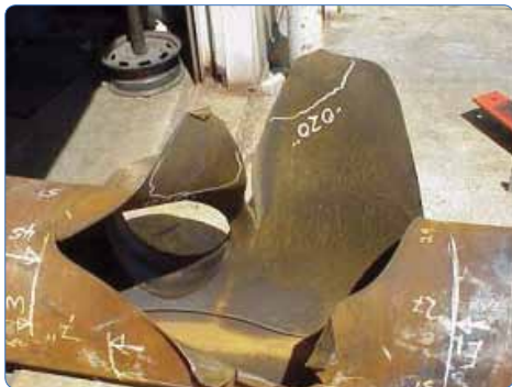
Carbon steel piping has failed catastrophically from FAC
