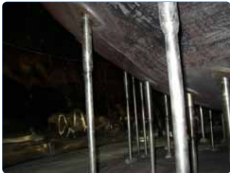
Bottom mounted Instruments present a challenge for mechanical Integrity assessment.
