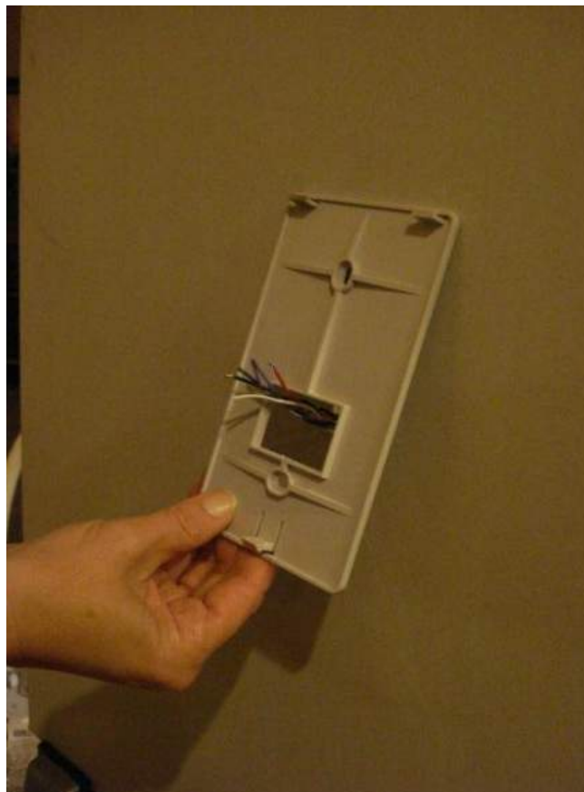
Figure 3 Replace with new sensor mounting plate
