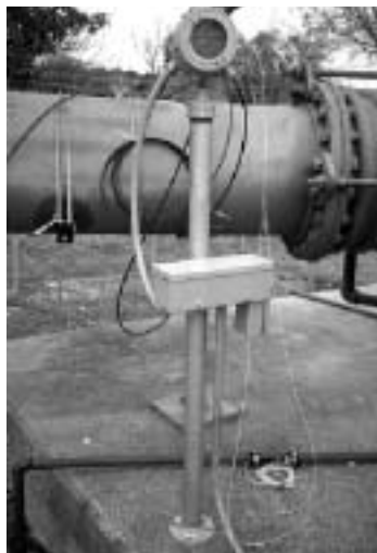
XMT868 clamp-on ultrasonic flowmeter installation
