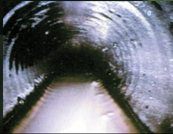
Service Water Line – Baseline Inspection
