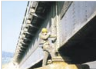
▼ Structural survey of a steel box-girder railroad bridge
