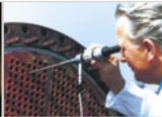
▼ Inspecting a tubed heat exchanger
